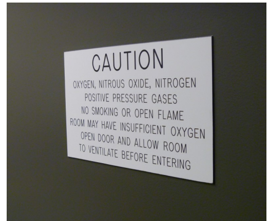
Figure 19. Equipment Room Wall Plate.
